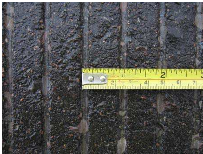
Figure 14(a): Example of a properly grooved runway. The grooves are 3 mm wide, 4 mm deep and 25 mm apart.
