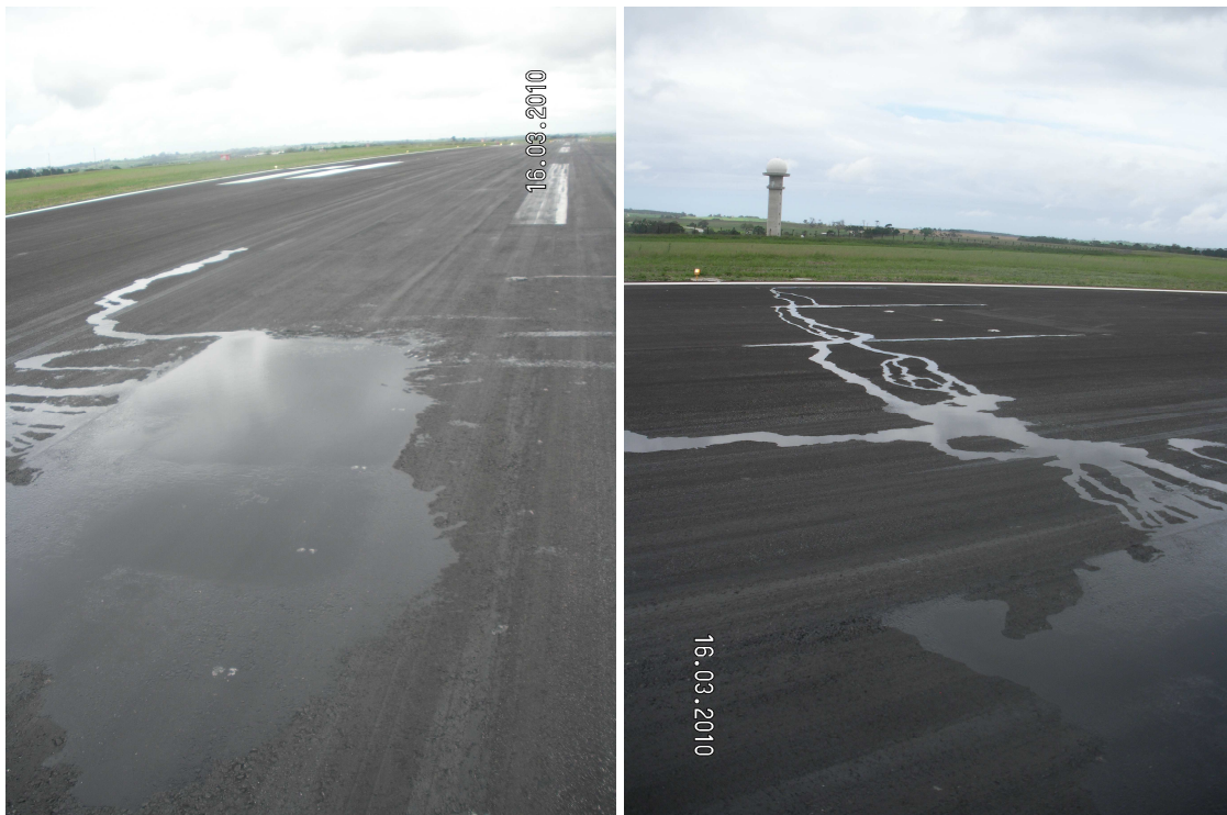
Figure 24: The puddle of water on the runway and the subsequent runoff to the left of the runway.
