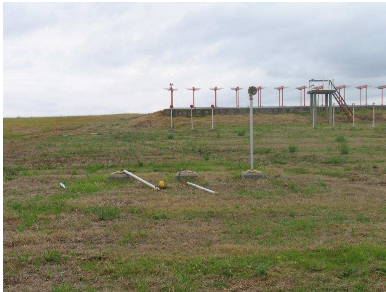
Figure 35: The ILS localiser antenna and damaged approach lights.
