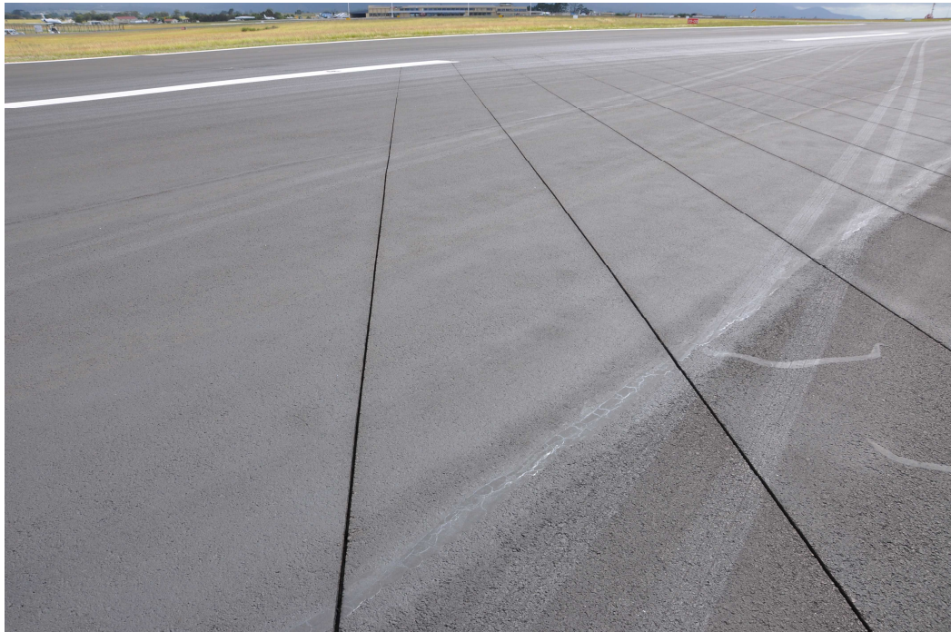
Figure 12: The slots cut into the runway surface at George aerodrome.
