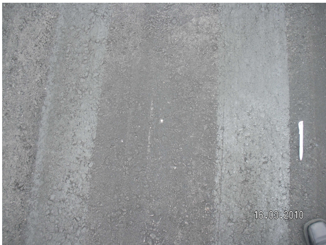
Figure 46: The texture of the tyre markings and adjacent runway surface
