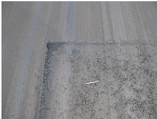
Figure 23(a): A milled area on the runway.
