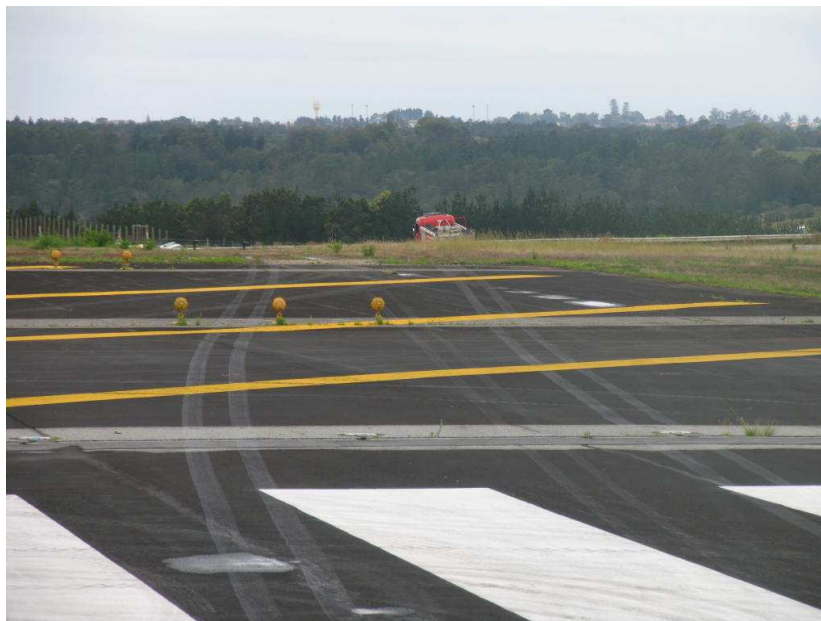
Figure 34: The tyre tracks indicating where the aircraft overran the runway surface onto the stop-way.
