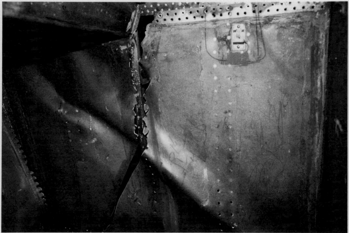
View of Centre Spar Web Forming Rear of Auxiliary Tank Bay
