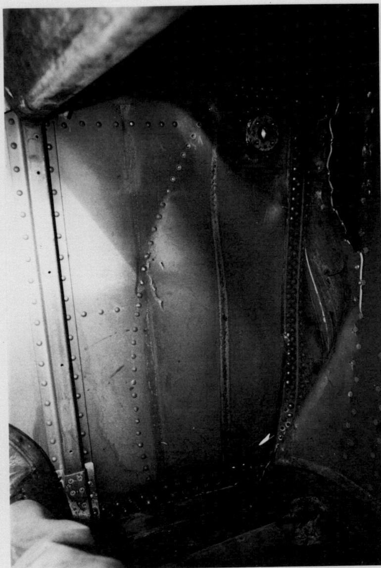
View of Front Spar Web from Inside Auxiliary Tank Showing Sheared Rivets, Buckles and Torn Rib
