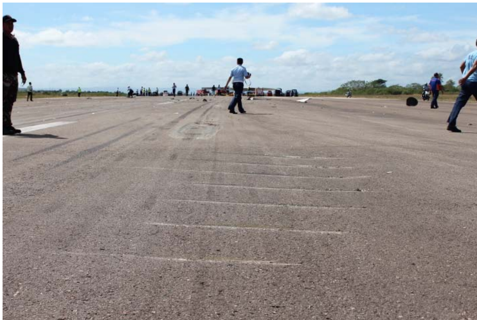
Figure 13: The propeller scratch marks
