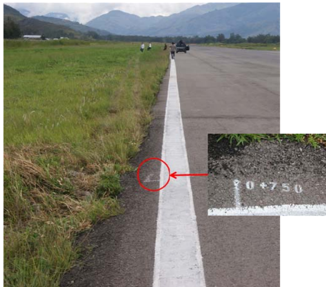
Figure 6: The mark of left main wheel off the runway
