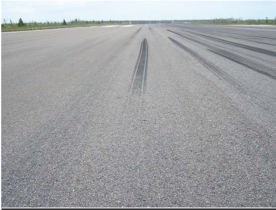
Signature marks of touchdown point on Runway 06 approximately 8,100 feet from the threshold of the 11,000 feet runway.
