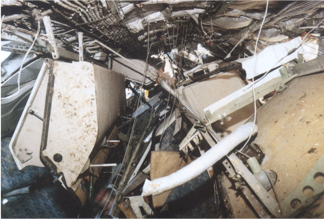
Figure 6a View of passenger cabin looking aft
