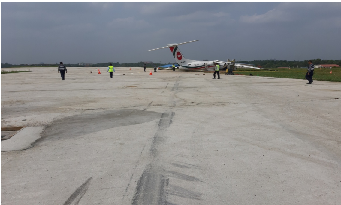
Figure (15) Wheel tracks and propeller striking marks on the overrun
