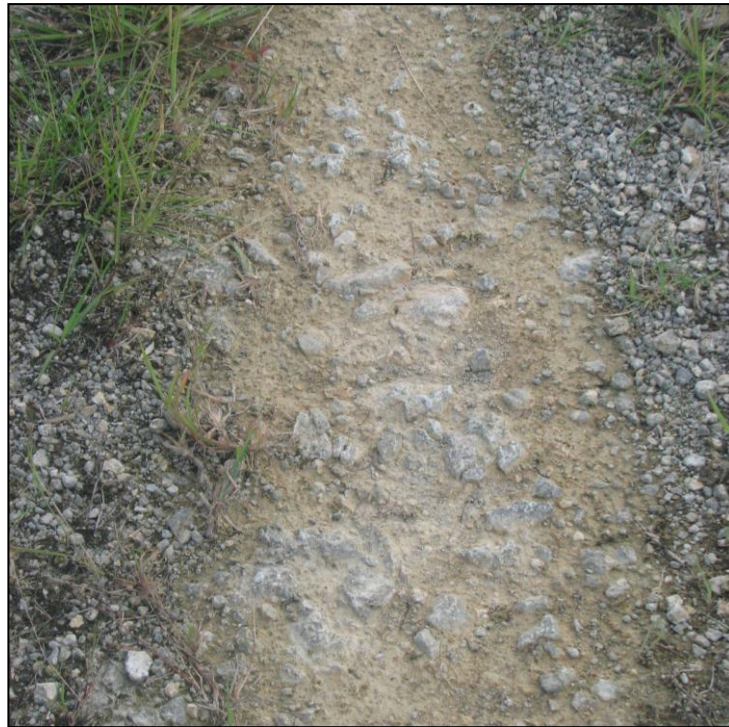
Figure 12: Removal of the small stones and dust from the landing tyre tracks
